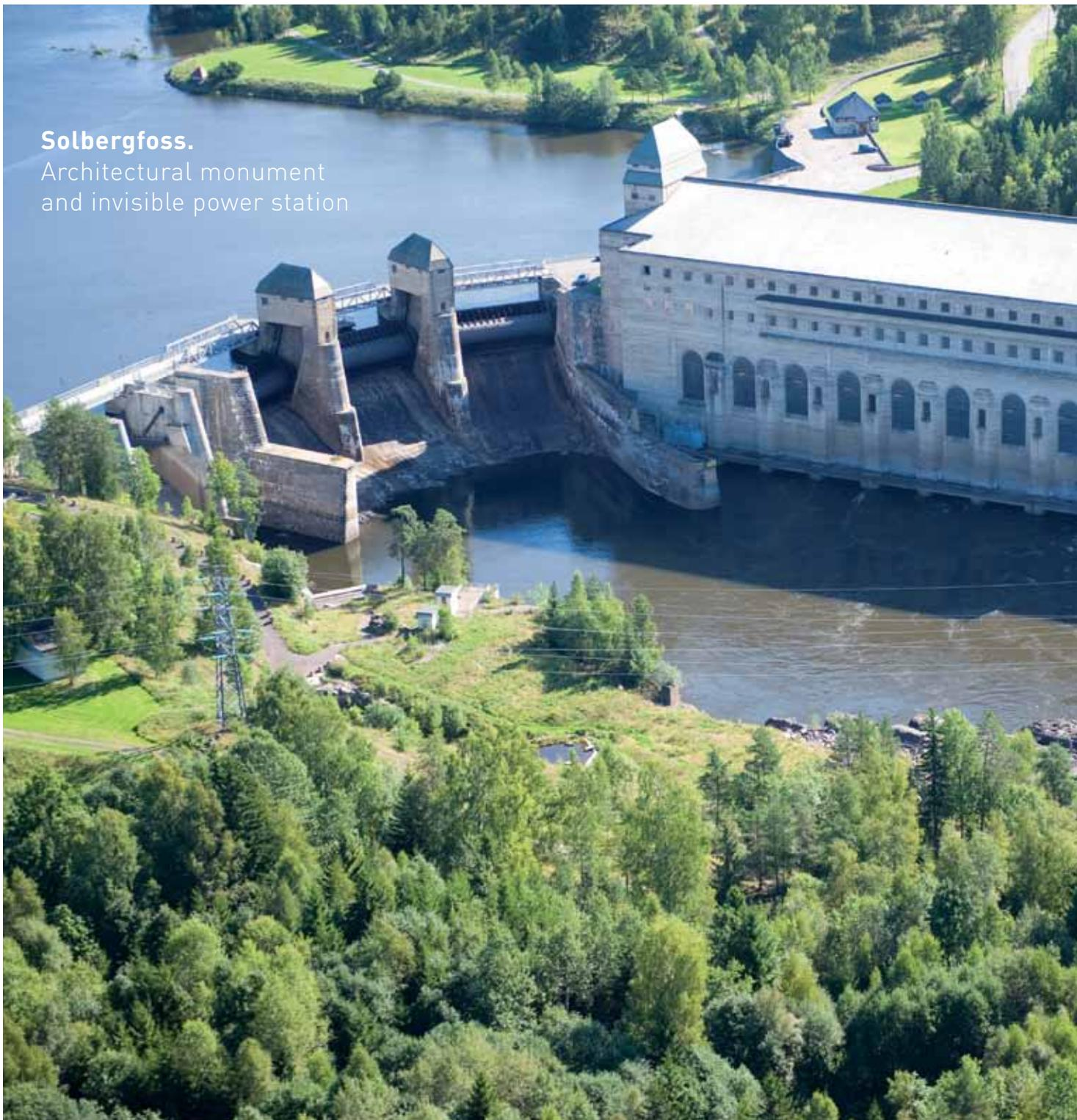
Solbergfoss is a hydraulic power plant. This means the turbines are run by power produced by the huge through-flow of water rather than by high waterfalls. The stations currently consist of two different power plants that were built at different times and based on different cultures.
