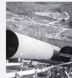
The first development project left the inlet pipes visible.
