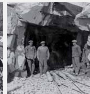
Inlet tunnels and power stations were also built inside mountains.
